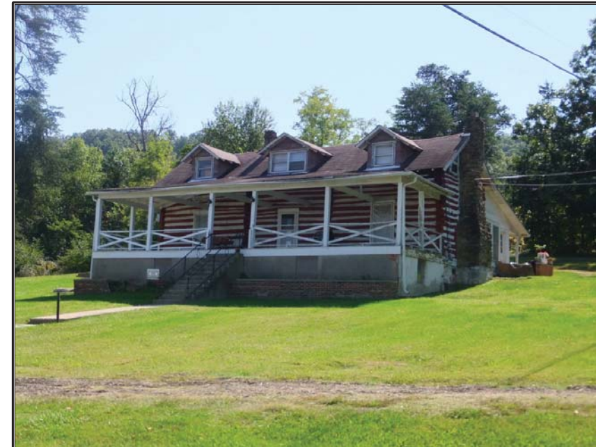
Figure 28. South-southeasterly view of log structure at 2500 South Park Road (CRA-2).
