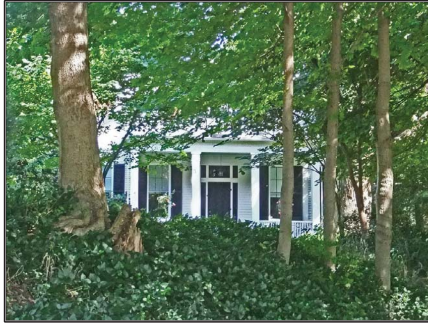
Figure 19. North-northeasterly view of Allison-Barrickman House (JF 563).
