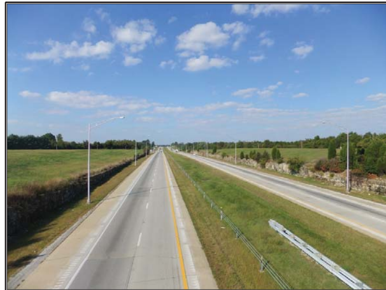
Figure 29. West-southwesterly overview of I-265 at Billtown Road.
