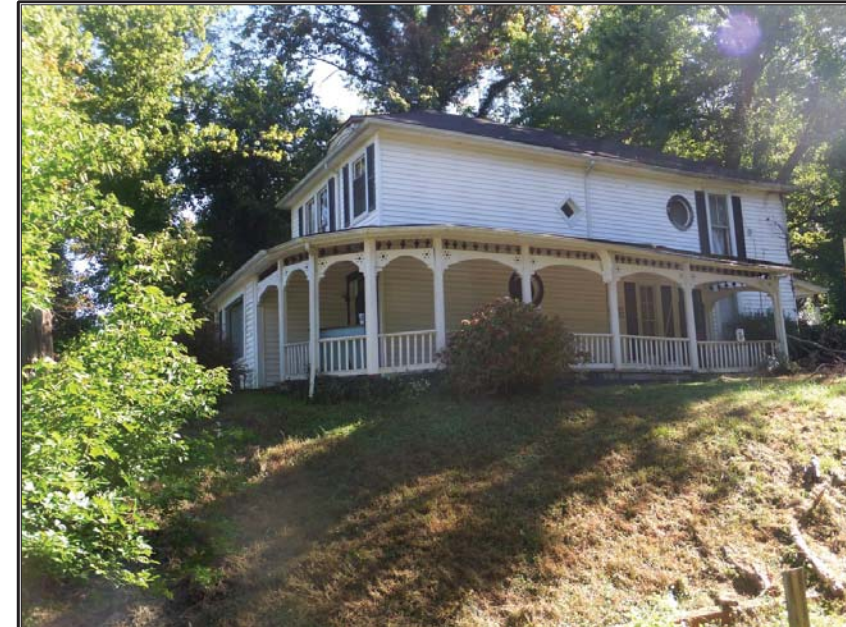
Figure 18. East-northeasterly view of Merriwether House (JF 690).
