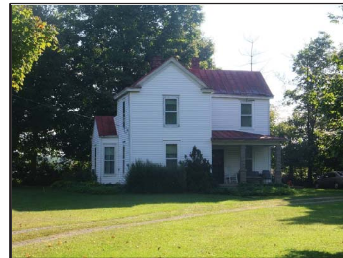
Figure 24. Southeasterly view of potentially eligible house at 3813 Hopewell Road (JF 1741).
